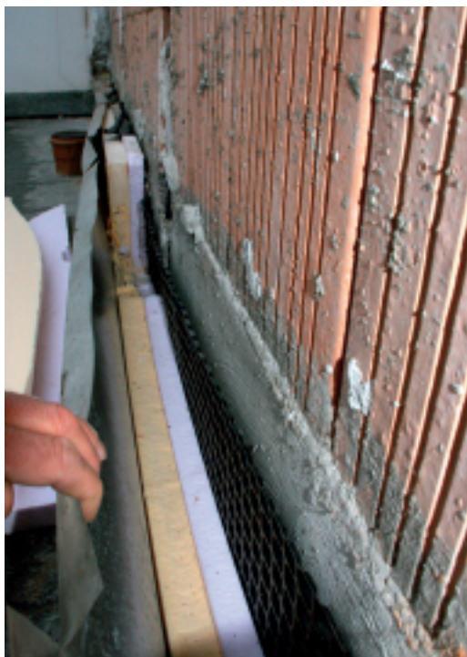
Correct installation is the only way to prevent radon-containing soil gas from rising and entering
