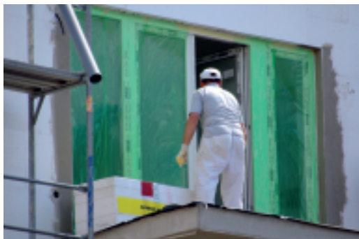
Retrofitting thermal insulation affects the air-tightness of the building envelope
